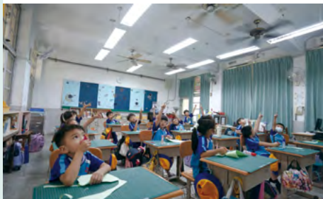
Campus LED Installation Projects
